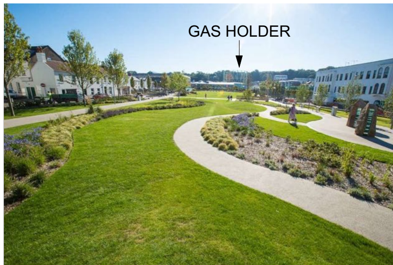
1. View across park of Gas Holder
