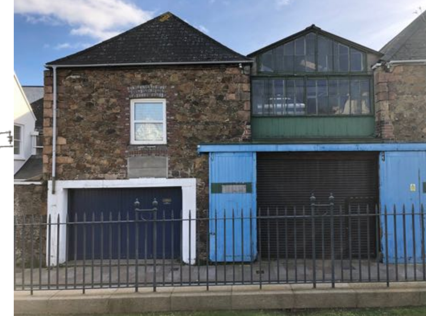
The Workshop, Tunnell Street
