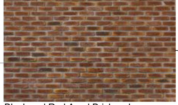
Black and Red Aged Brickwork
