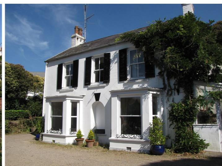
Existing Photograph of Western Elevation
