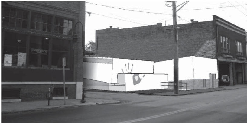
view of entrance
