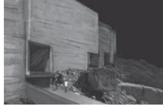
re-entry of house to washroom
