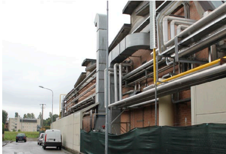
SITE CONDITION: THE INDUSTRIAL FACADE
