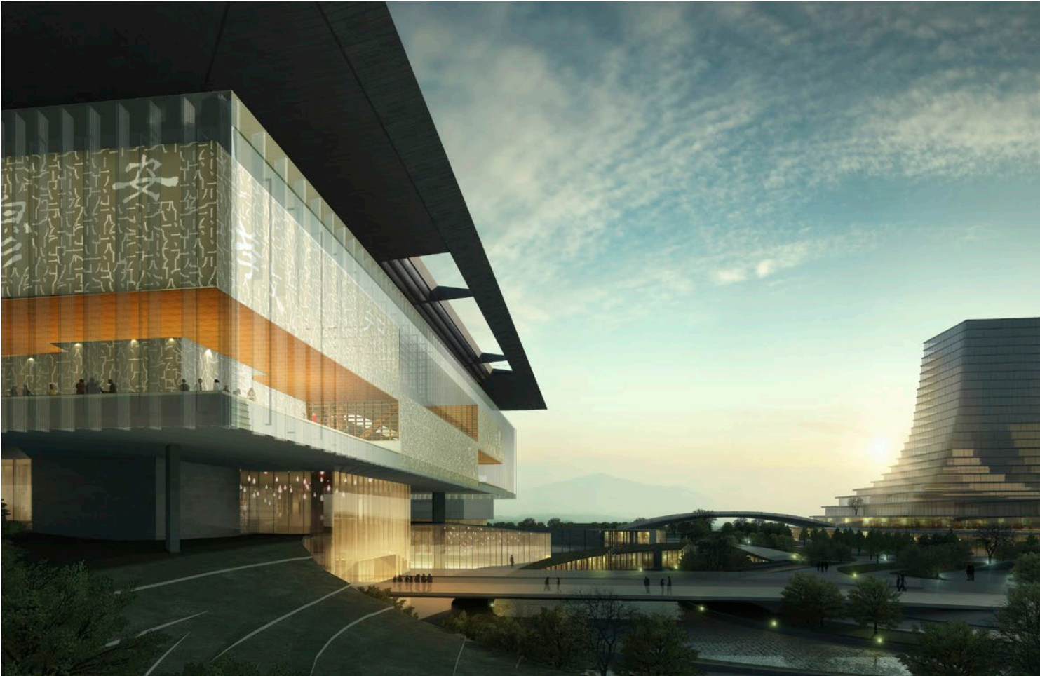
SOUTH EAST CORNER LOOKING AT THE ENTRANCE AND FACADE
