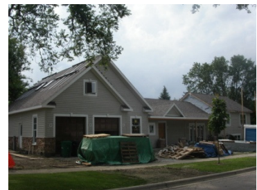
Currently Under Construction
