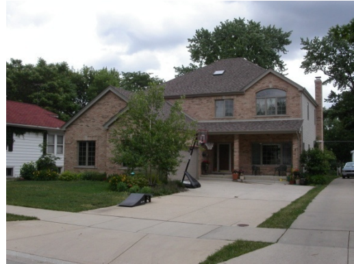
204 Columbia - Elmhurst, IL New Construction
