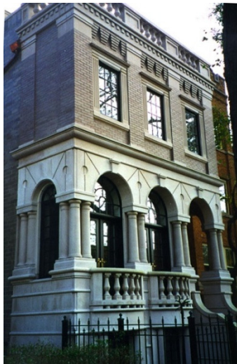
2360 Dayton – Chicago, IL New Construction
