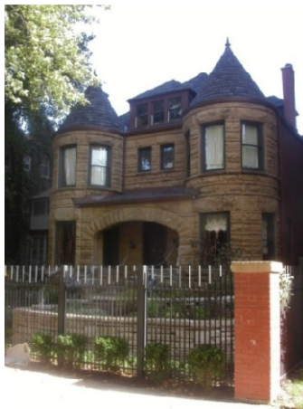
5522 Hyde Park Blvd. – Chicago, IL Complete Interior Remodeling
