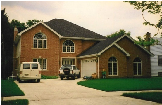
177 Fremont Street - Elmhurst, Illinois New Construction
