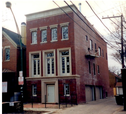
2544 Wayne Street – Chicago, IL New Construction
