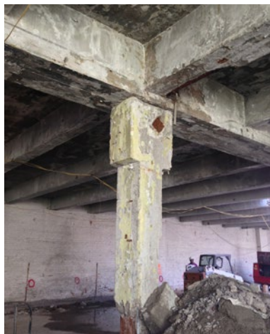
| existing concrete encased steel column
