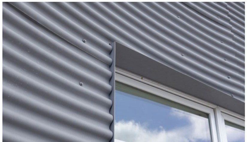
| detail photos of zinc rain screen
