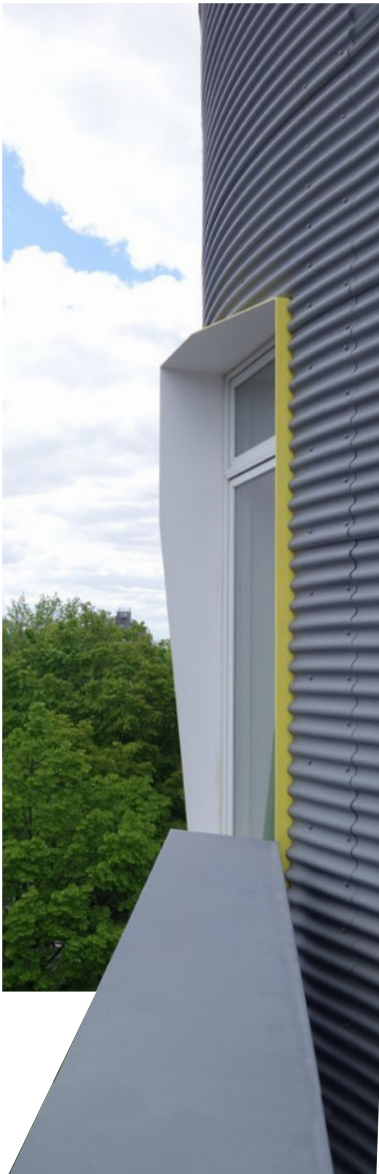
| detail photos of zinc rain screen
