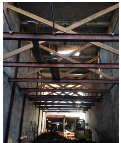
| new steel and temporary wood bracing
