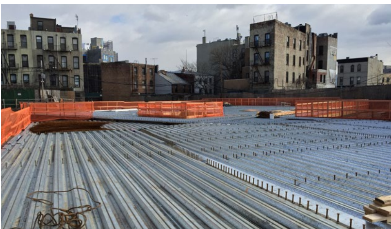
completed decking at ground floor
