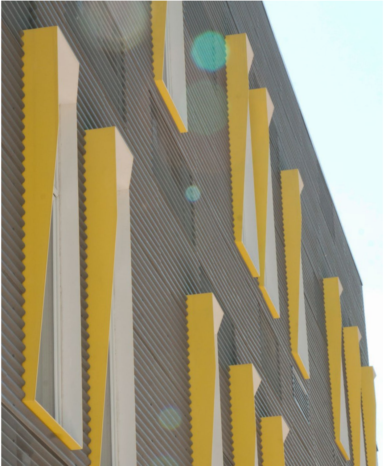
| corrugated zinc facade punctuated by joy yellow "eye-lid" solar shades
