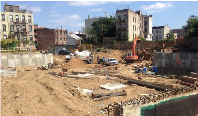
preliminary foundation work and excavation
