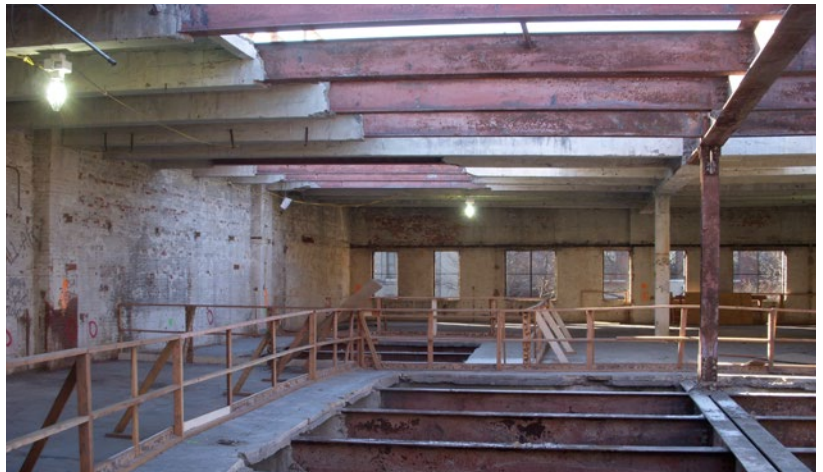
| demolition of existing slab to make way for proposed central courtyard
