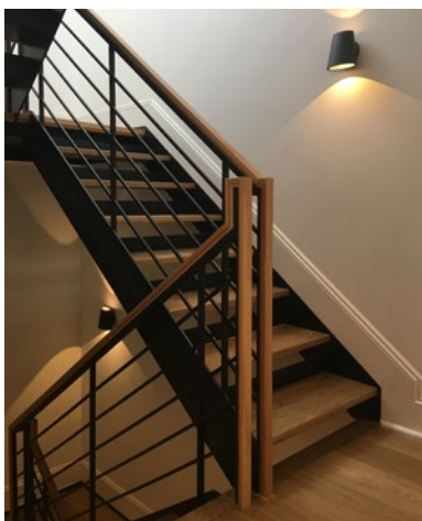
| detailing of new custom wood & steel staircase
