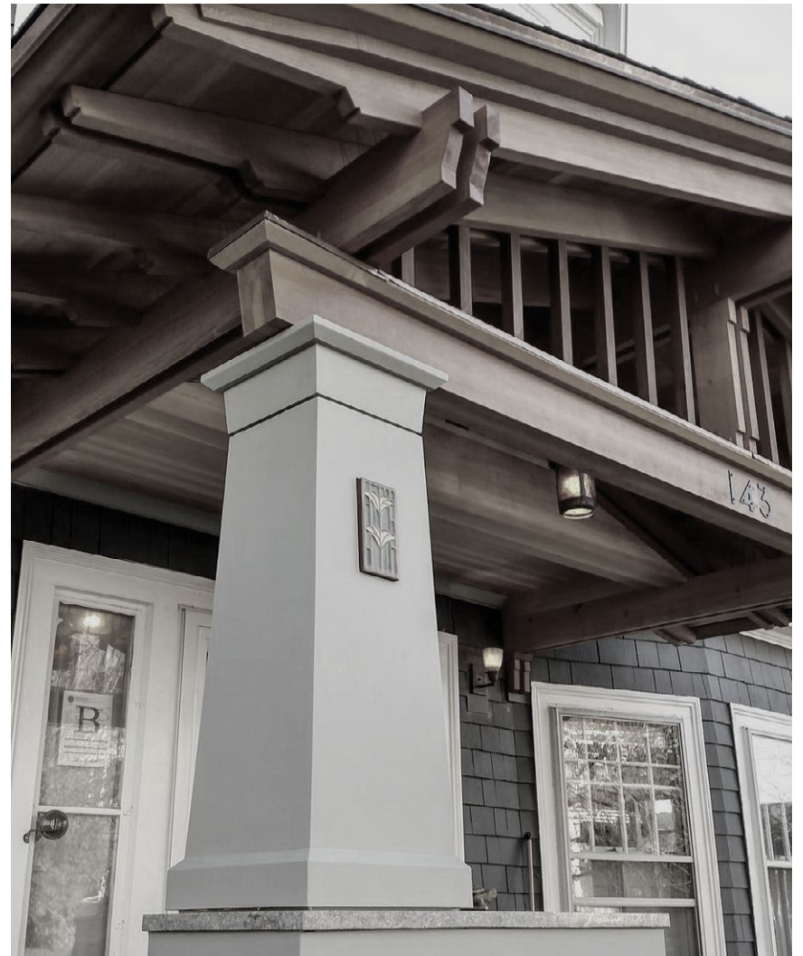
Fir timber framed porch with marble top pedestals
