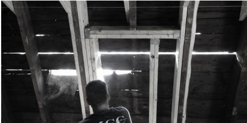
Skylight installation in third floor remodel
