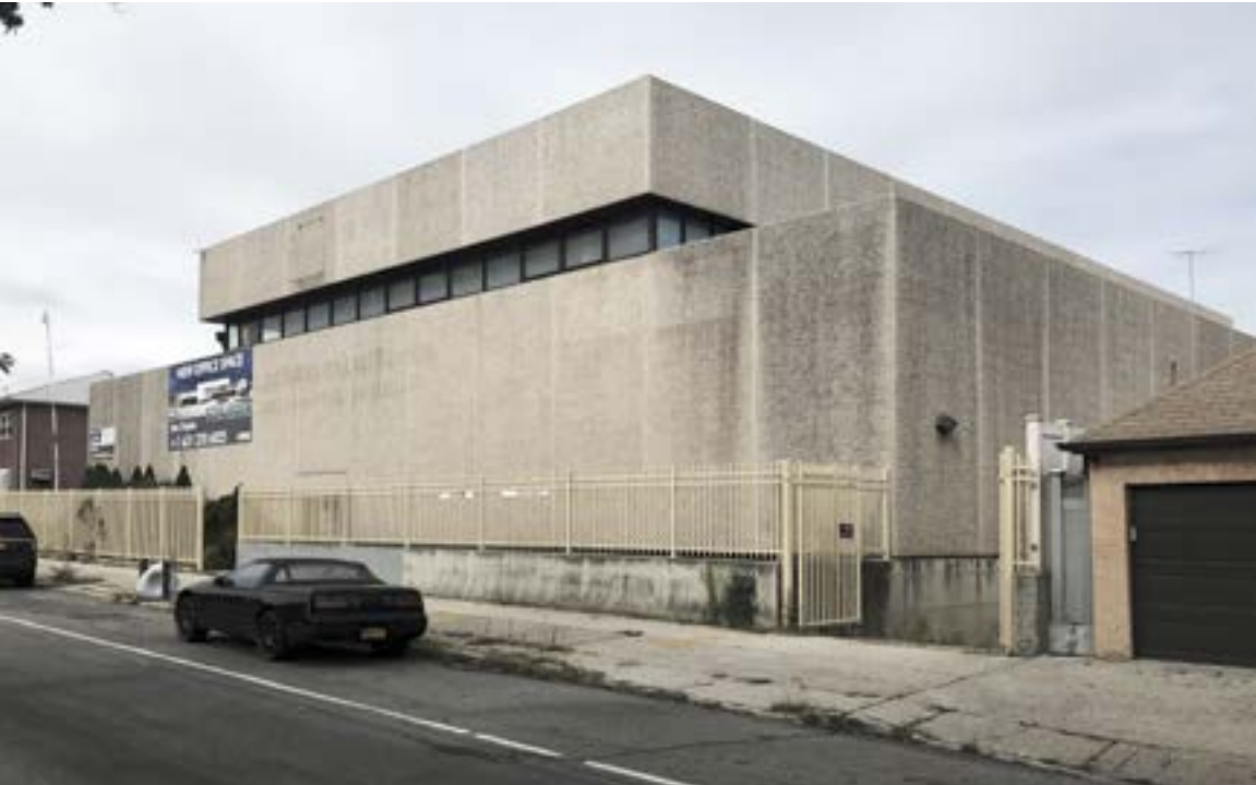
PREVIOUS WOODHAVEN BLVD (WEST) FACADE
