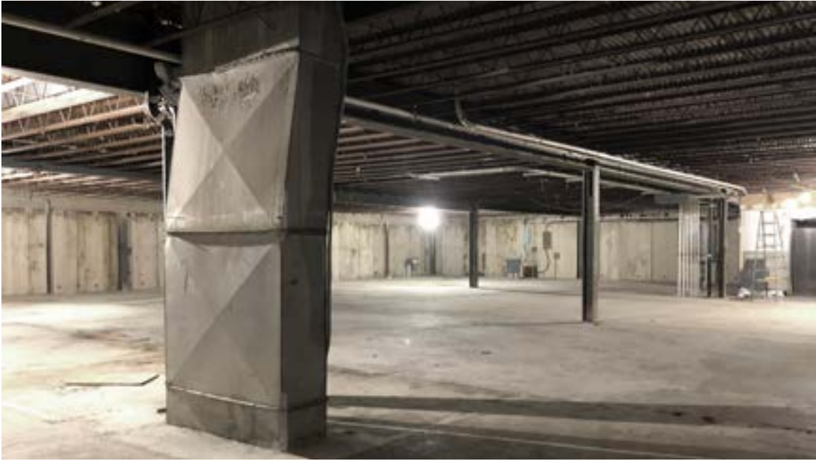
PREVIOUS FIRST FLOOR (NO WINDOW, FULLY ENCLOSED BY PRECAST PANEL)
