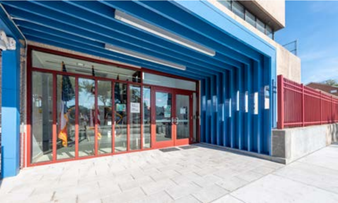
NEW CANOPY AT WOODHAVEN BLVD (WEST) FACADE
