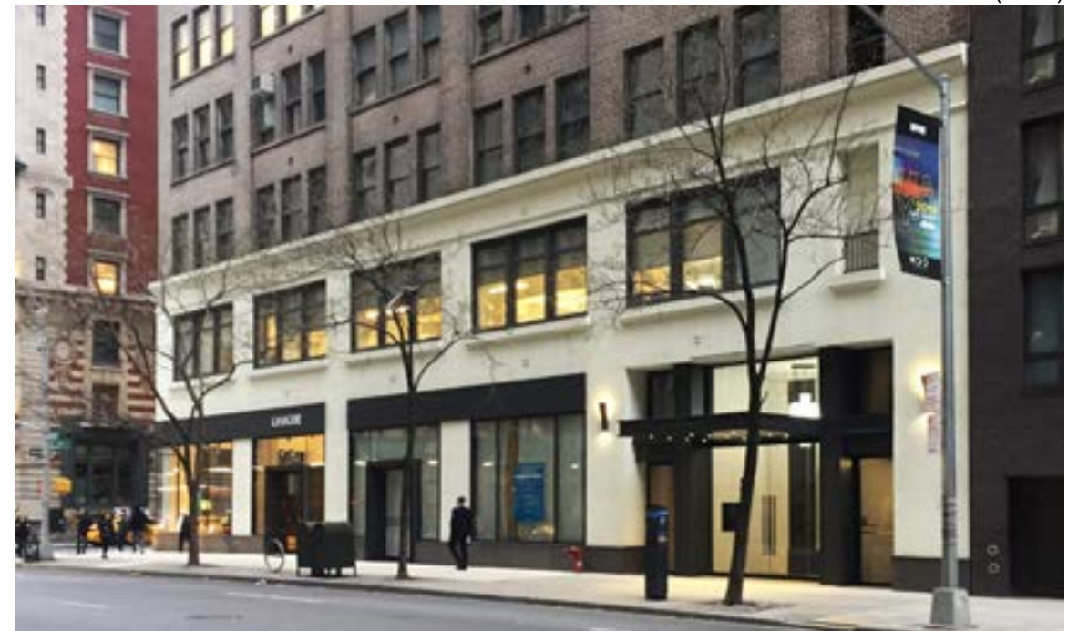
NEW STOREFRONT MADISON AVE VIEW (2019)
