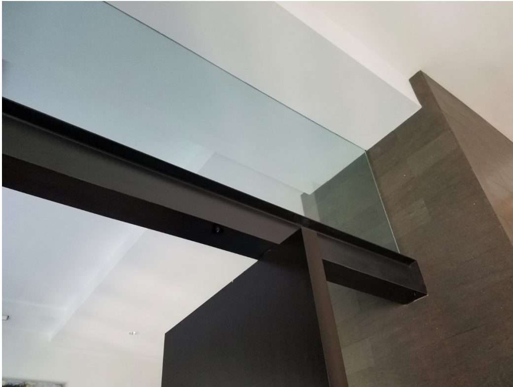
PIVOT DOOR, BEAM & TRANSOM DETAIL
