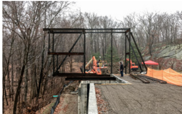
STRUCTURAL STEEL FOR CANTILEVER
