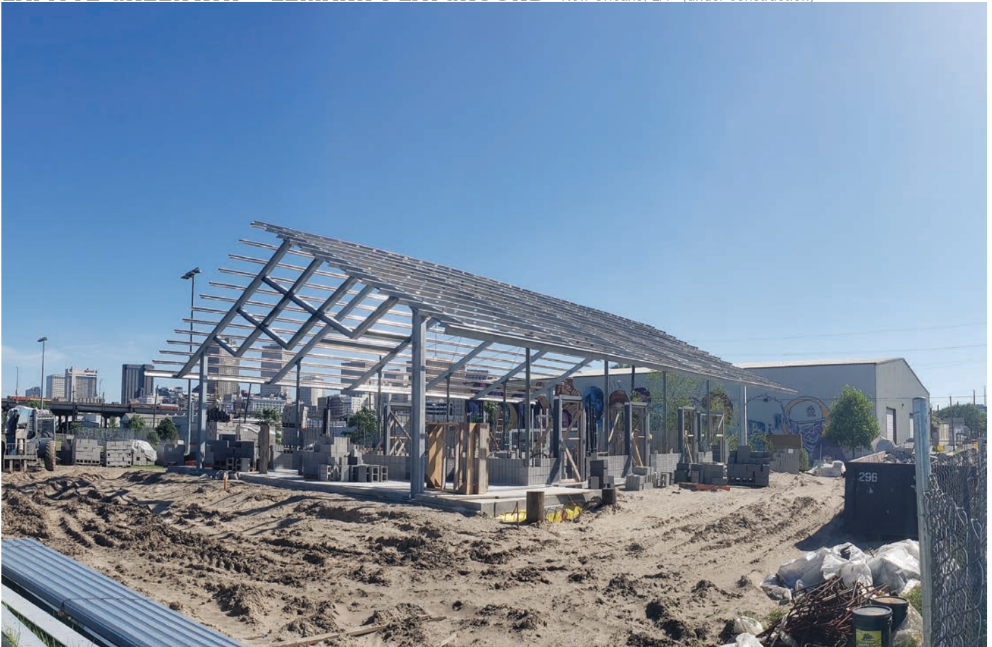
LAFITTE GREENWAY - LEMANN PLAYGROUND New Orleans, LA (under construction)
