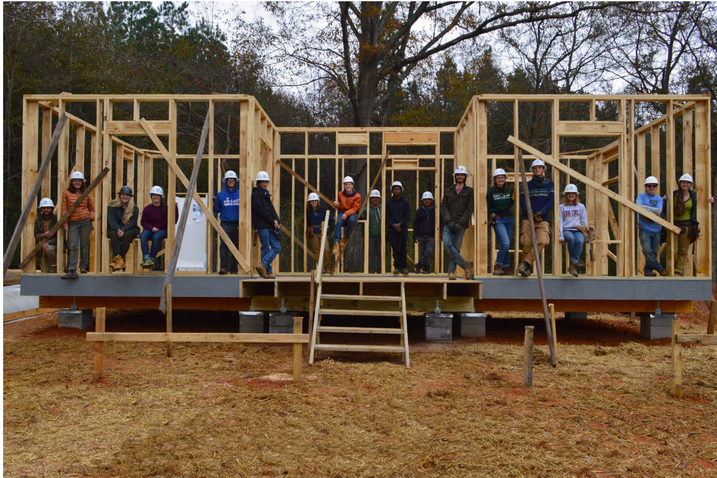
At the end of the Fall Semester, the student team completed construction on the house's footings, floor platform, and exterior walls. (Photo Credit: Yoon Dong Kyu)
