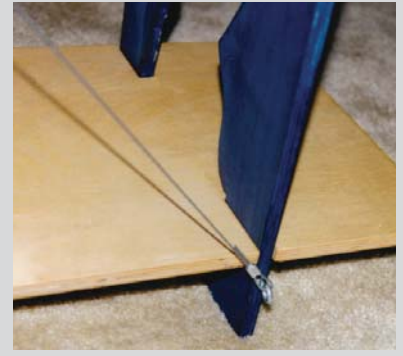
Minimum material display: The fish inspired cutout allows the shelves to rotate and lock into place and support all loads. Steel cables with turnbuckles provide lateral stability. The five equal pieces of a 5'x 5' sheet of Baltic birch plywood contrasts finishes of natural tung oil and a denatured alcohol based stain.
