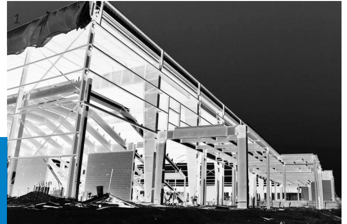
Construction Photos: Main steel truss column members (Gatheing Pavilion/Bell-Tower)
