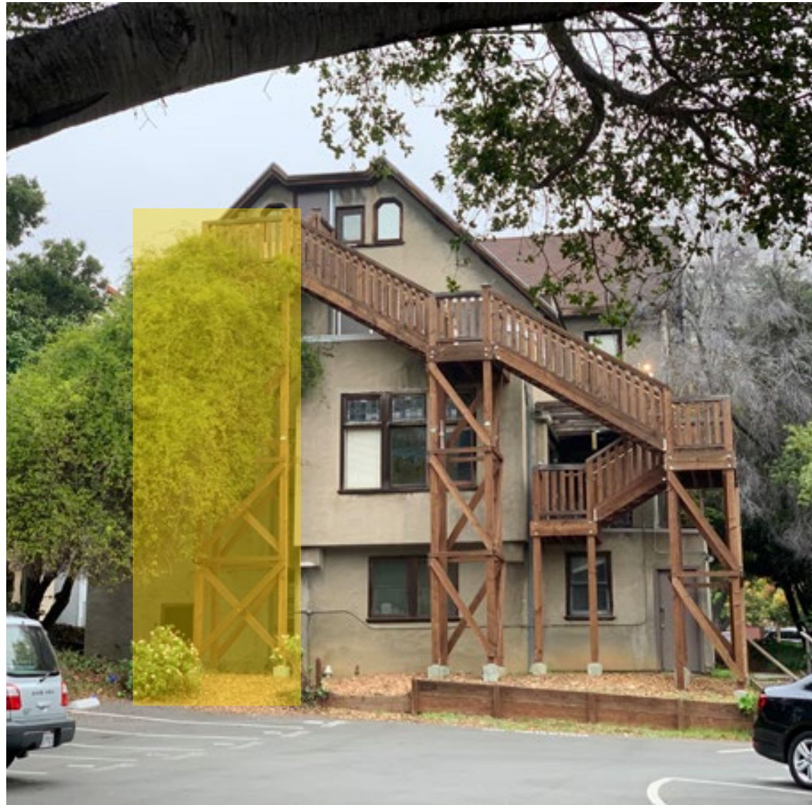
Photograph of the east elevation. Shaded yellow region indicates location of the new elevator tower addition.
