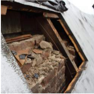
PROBE TO DETERMINE FRAMING
