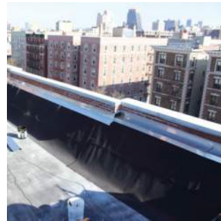
NEW PARAPET COPING AND FLASHING
