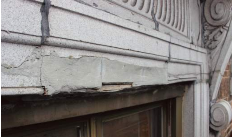
DEFECTIVE TERRA-COTTA LINTEL
