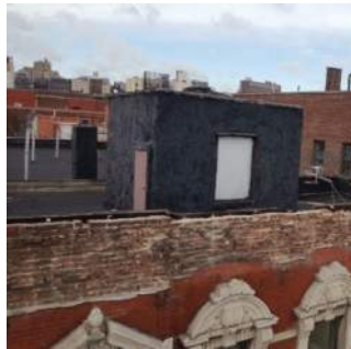
PARAPET AFTER CORNICE REMOVAL
