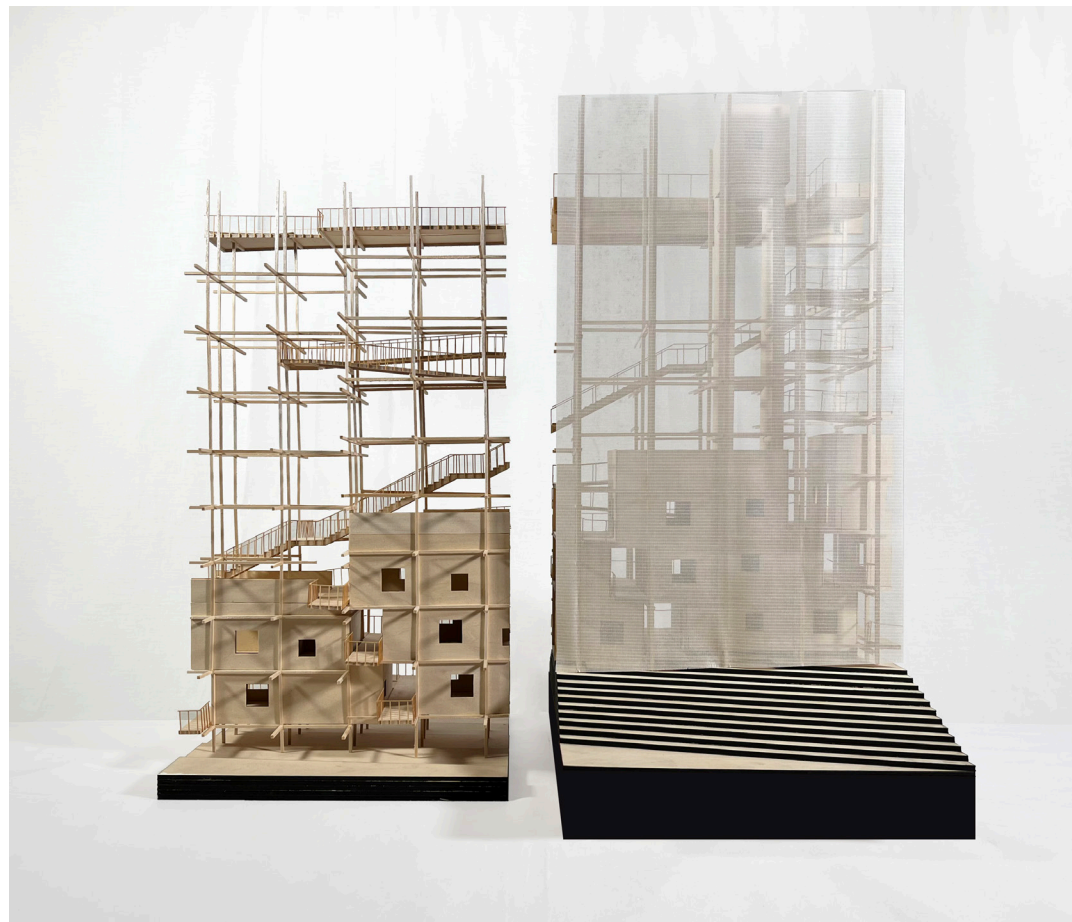
Above: A sectional model showing the way that the steel structure penetrates the CLT housing units. In a disaster event, the CLT is expected to be sacrificial, leaving the steel structure to support the refuge platform.
