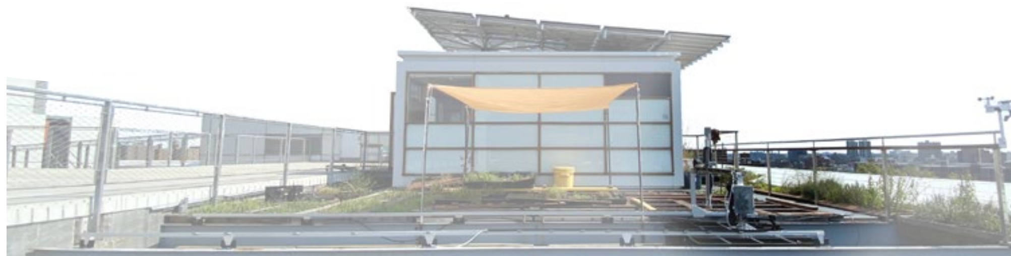
Site Photo upon Conclusion
