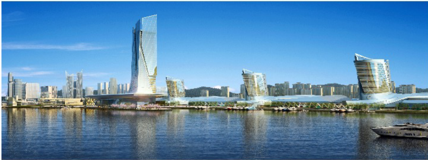
Dalian Convention Center Masterplanning | Hotel, Convention Center, Commercial and Residential Neighborhoods Schematic Design. Competition
