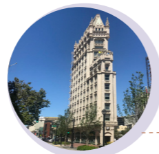
VIEW 1 Cathedral Building
