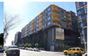
CROSBY (II) 685 S CATALINA ST LOS ANGELES, CA 90010 MULTI-FAMILY 8 STORY / 120 UNITS TYPE III OVER EXISTING PARKING GARAGE / JUNE 2020
