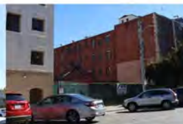
BLDG 23 738 S NORMANDIE AVE LOS ANGELES, CA 90005 MIXED-USE / MULTI-FAMILY / RETAIL 7 STORY / 44 UNITS GROUND-UP / UNDER CONSTRUCTION
