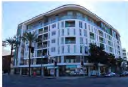
NOVA 3980 WILSHIRE BLVD LOS ANGELES, CA 90005 MIXED USE / MULTI-FAMILY / RETAIL 7 STORY / 228 UNITS GROUND-UP / NOVEMBER 2020
