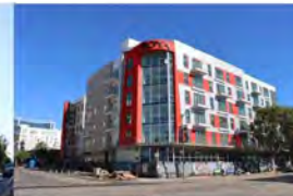
NOVA 760 SERRANO AVE LOS ANGELES, CA 90005 MIXED USE / MULTI-FAMILY / RETAIL 6 STORY / 357 UNITS GROUND-UP / UNDER CONSTRUCTION
