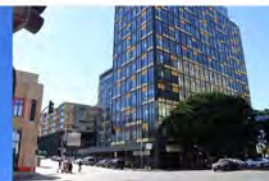
CROSBY (I) 3350 WILSHIRE BLVD LOS ANGELES, CA 90010 MIXED-USE / MULTI-FAMILY / RETAIL 12 STORY / 216 UNITS ADAPTIVE RE-USE / SEPTEMBER 2020
