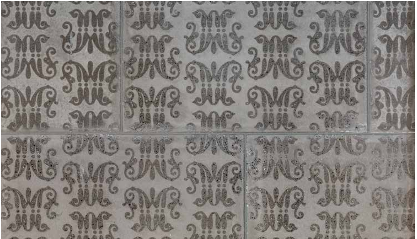
Photo of Marist Steel Plant Close-Up Photo of Precast Panels with Decorative Marist "M" Logo
