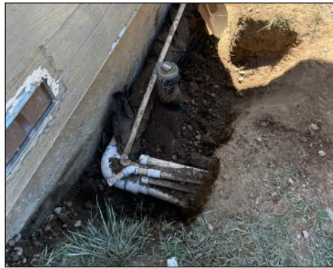
Digging & Extending Plumbing Lines
