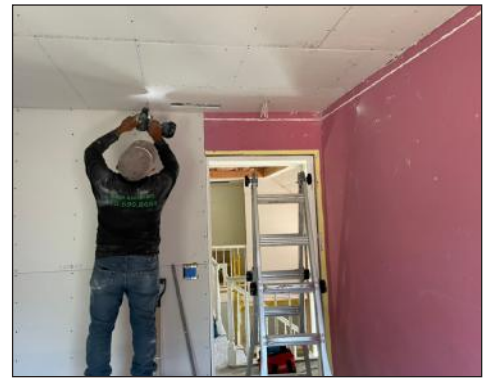
Installing Drywall Throughout the Home
