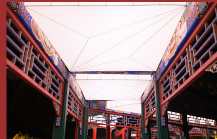
PARTY WATERSIDE PAVILLIONS
