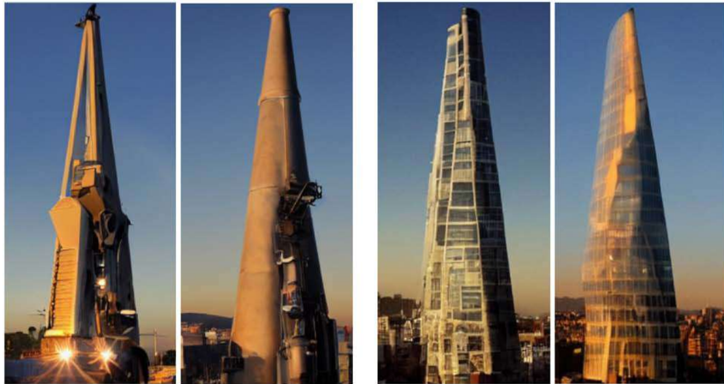
“Architecture is dominated by the food industry and exaggerated in its response to the building structure, with a large number of mechanical structures exposed to the air.”
