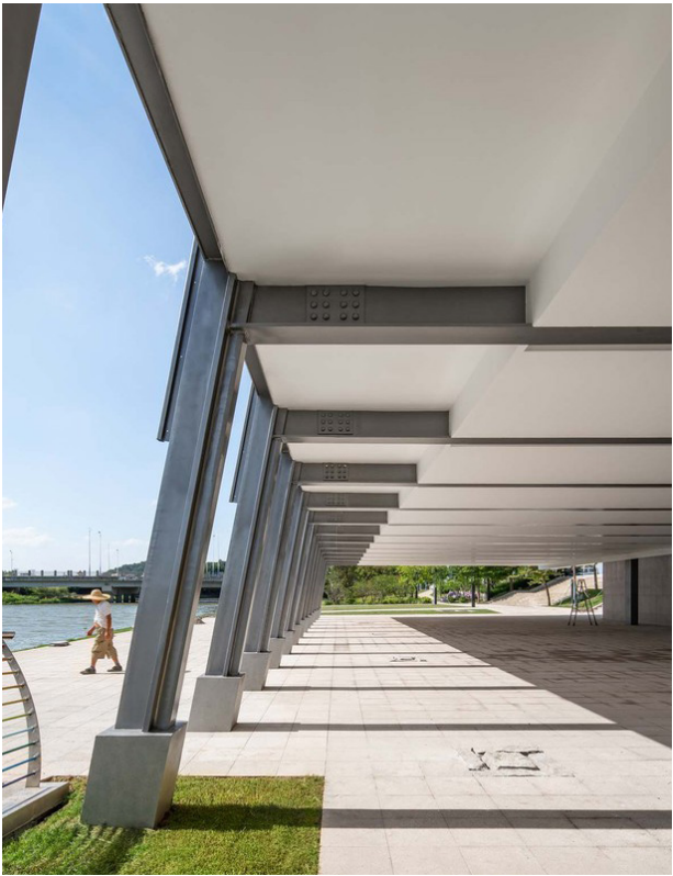
Suspended floor avoids the original walkways
