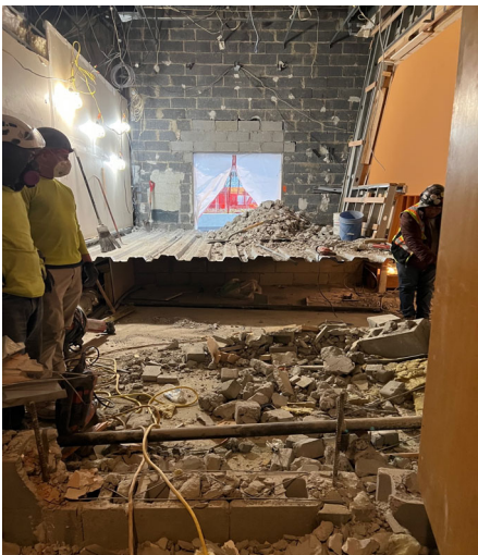
Demolition 50% raised floor ex PDR
