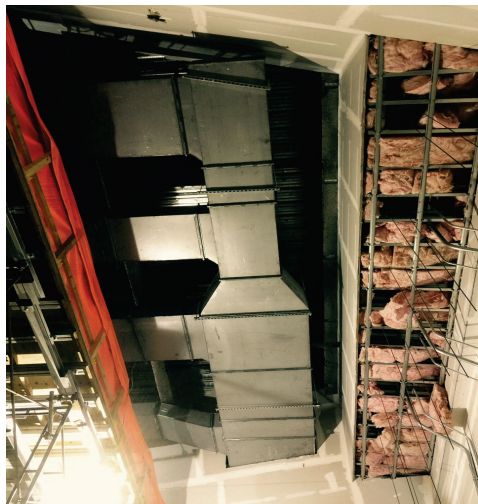
10 ph (06-21-2017) SA duct insatlled inside the Theater as per revised layout
