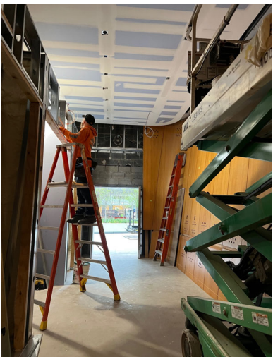
Construction Plaza Lobby
