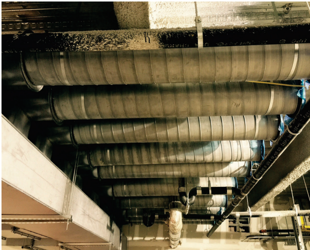
2 ph ((06-28-2017) SA ducts installed as per revised layout.
