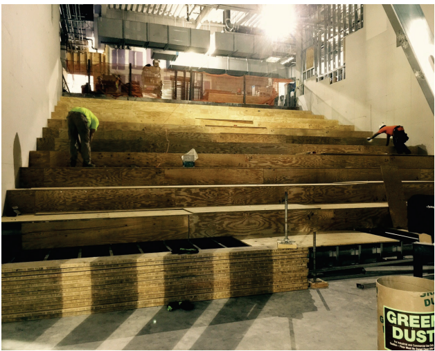
12 ph (05-19-2017) Theater seating work in progress.
