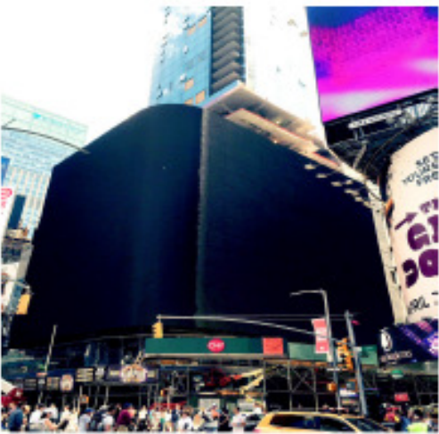
Fig. 2 Progress exterior (photo by M.Rengan)
