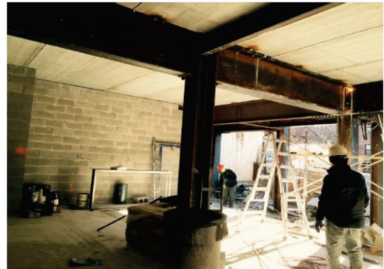
First Floor – Cross Beams at First Floor Lobby & Beams at Storefront
