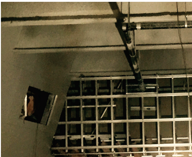
8 ph (05-30-2017) Theater - opening for SA Duct to be installed below pipe, inside the theater.
