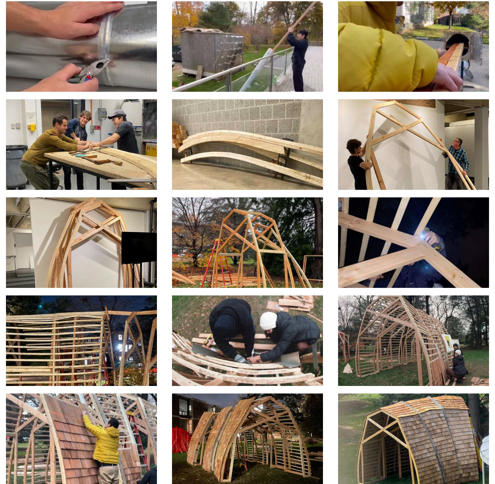
Fabrication of the Barn: Assembly of Steam Bender, Splicing 2x4s, Soaking of Wood, Steam Bending, Clamping, Shingling
