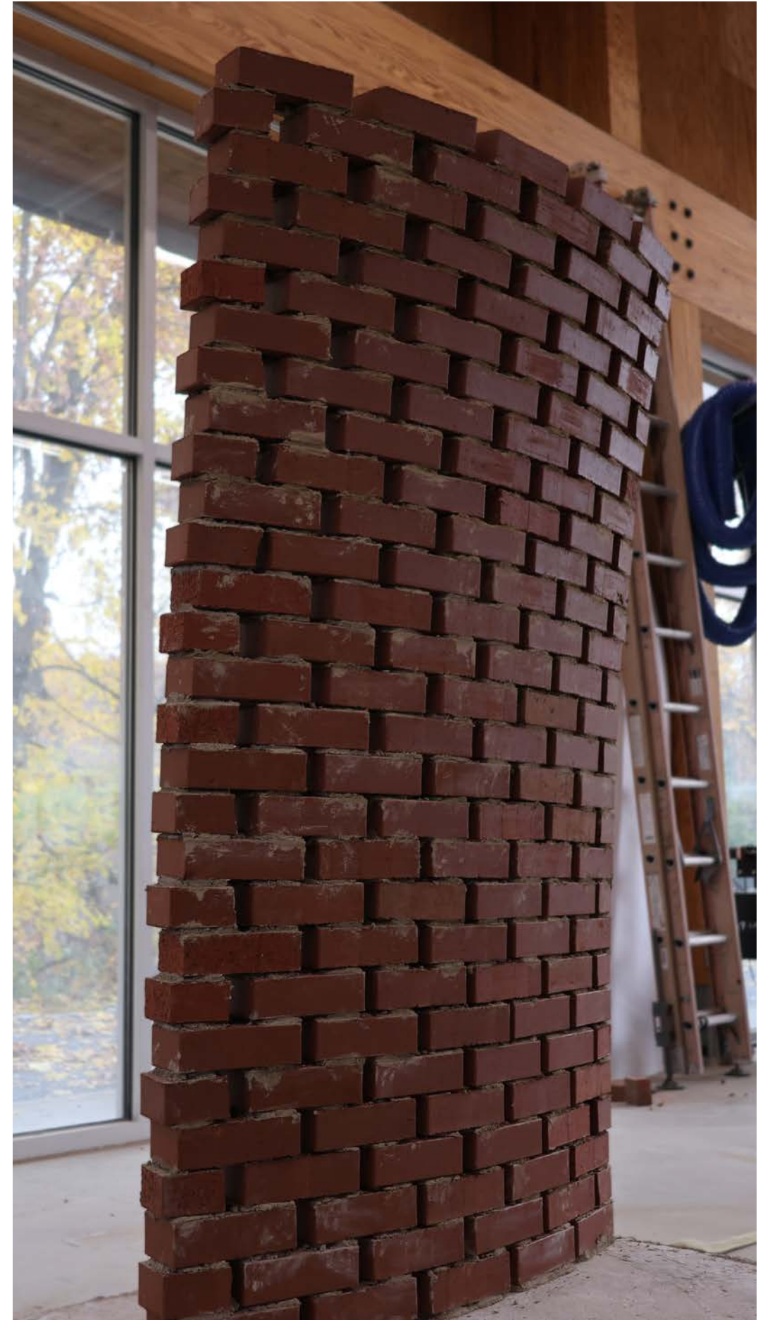
Structural Stability in the Brick Double-Curved Wall
