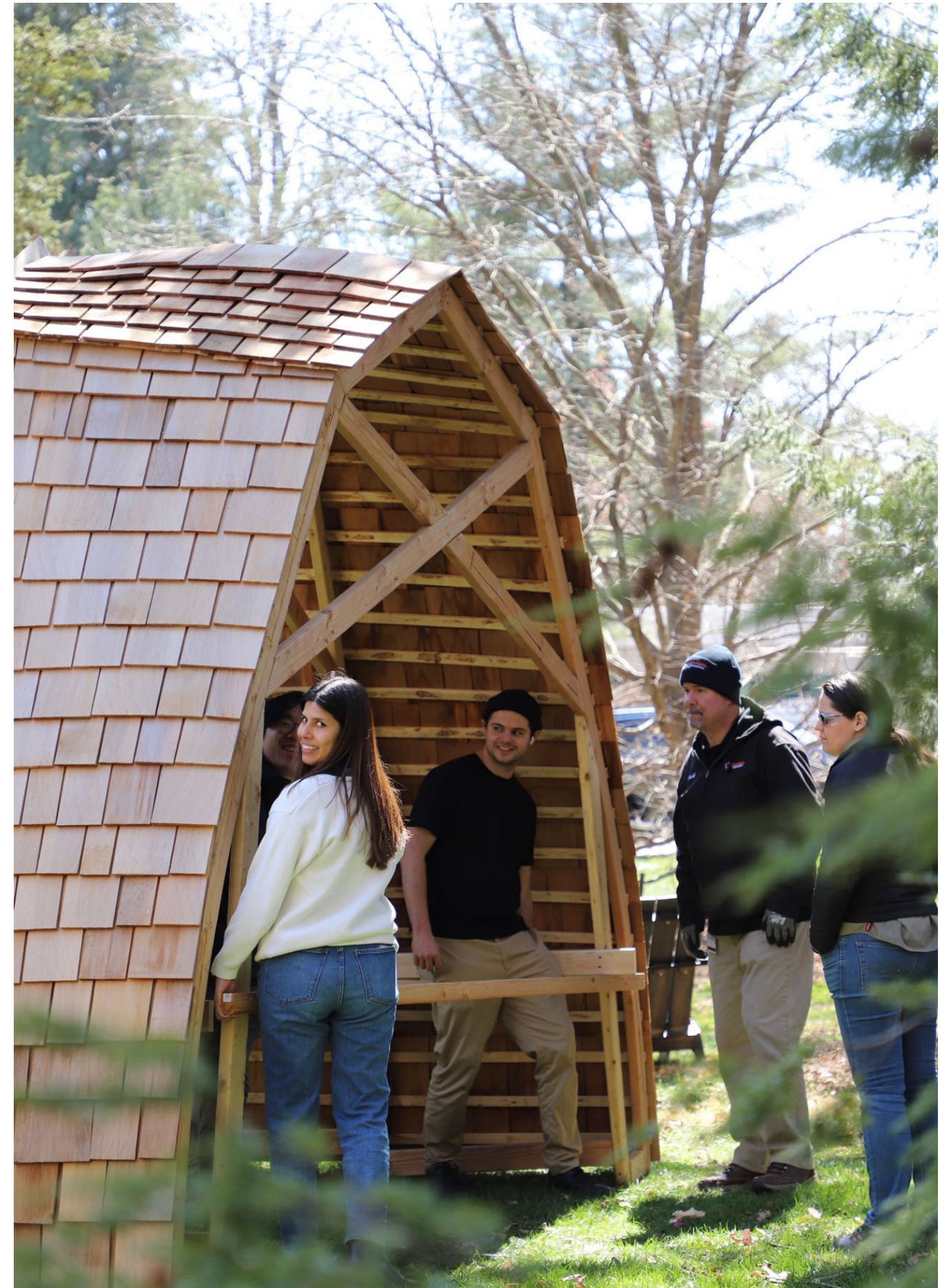
Attachment of 2x4 handles to Aid in Transport of Barn to Loading Truck
