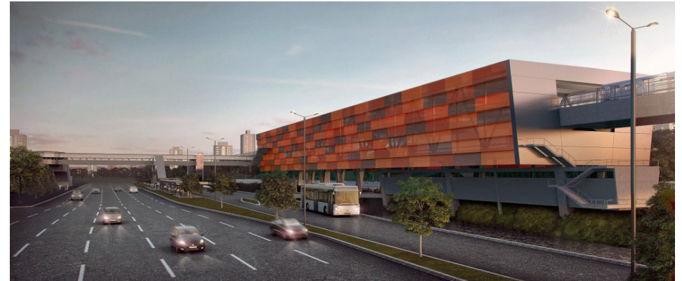
Detran Station - External view.
