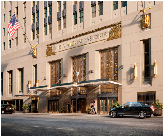
Storefront and Main Entrance - restoration associated to new architectural elements.
