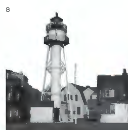
Coney Island Lighthouse Constructed: 1894, NJ Type: Terrestrial Height: 75' (SL: 0') Shape: Square Foundation: Steel Pile
