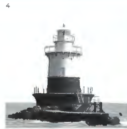
Old Orchard Shoal Constructed: 1893, NY Type: Aquatic Height: 35' (SL: 0') Shape: Conical Foundation: Calisson
