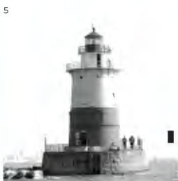
Robins Reef Lighthouse Constructed: 1839, NY Type: Aquatic Height: 45' (SL: 0') Shape: Conical Foundation: Calisson
