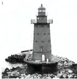
West Bank Lighthouse Constructed: 1910, NY Type: Aquatic Height: 55' (SL: 0') Shape: Conical Foundation: Calisson
