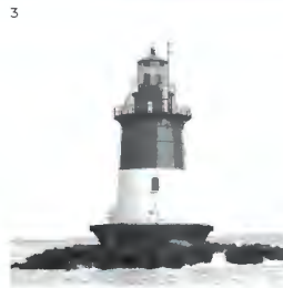
Romer Shoal Lighthouse Constructed: 1838, NY Type: Aquatic Height: 54' (SL: 0') Shape: Conical Foundation: Calisson
