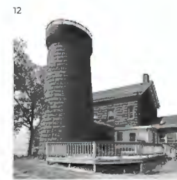
Prince's Bay Lighthouse Constructed: 1828, NY Type: Terrestrial Height: 40' (SL: 107') Shape: Conical Foundation: Rubblestone
