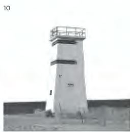
Breezy Point Lighthouse Constructed: 1914, NY Type: Terrestrial Height: 40' (SL: 0') Shape: Square Foundation: Concrete
