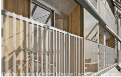
Double layered envelope system with operable polycarbonate panels.
