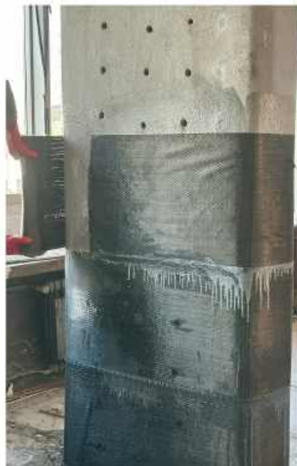
Carbon Fiber Wrapping Application
