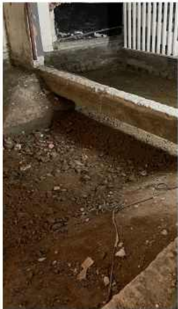
Raft Foundation Construction
