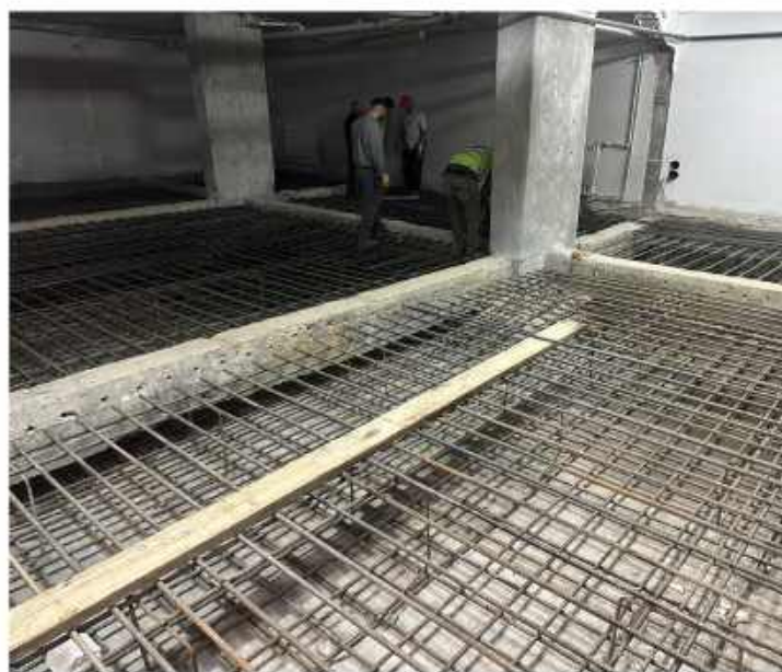
Raft Foundation Construction
