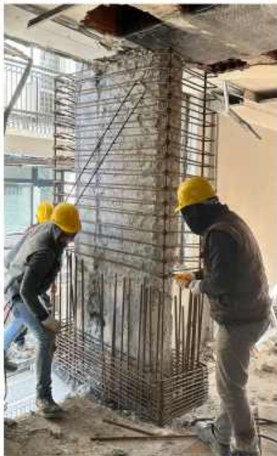
Reinforced Concrete Jacketing Production
