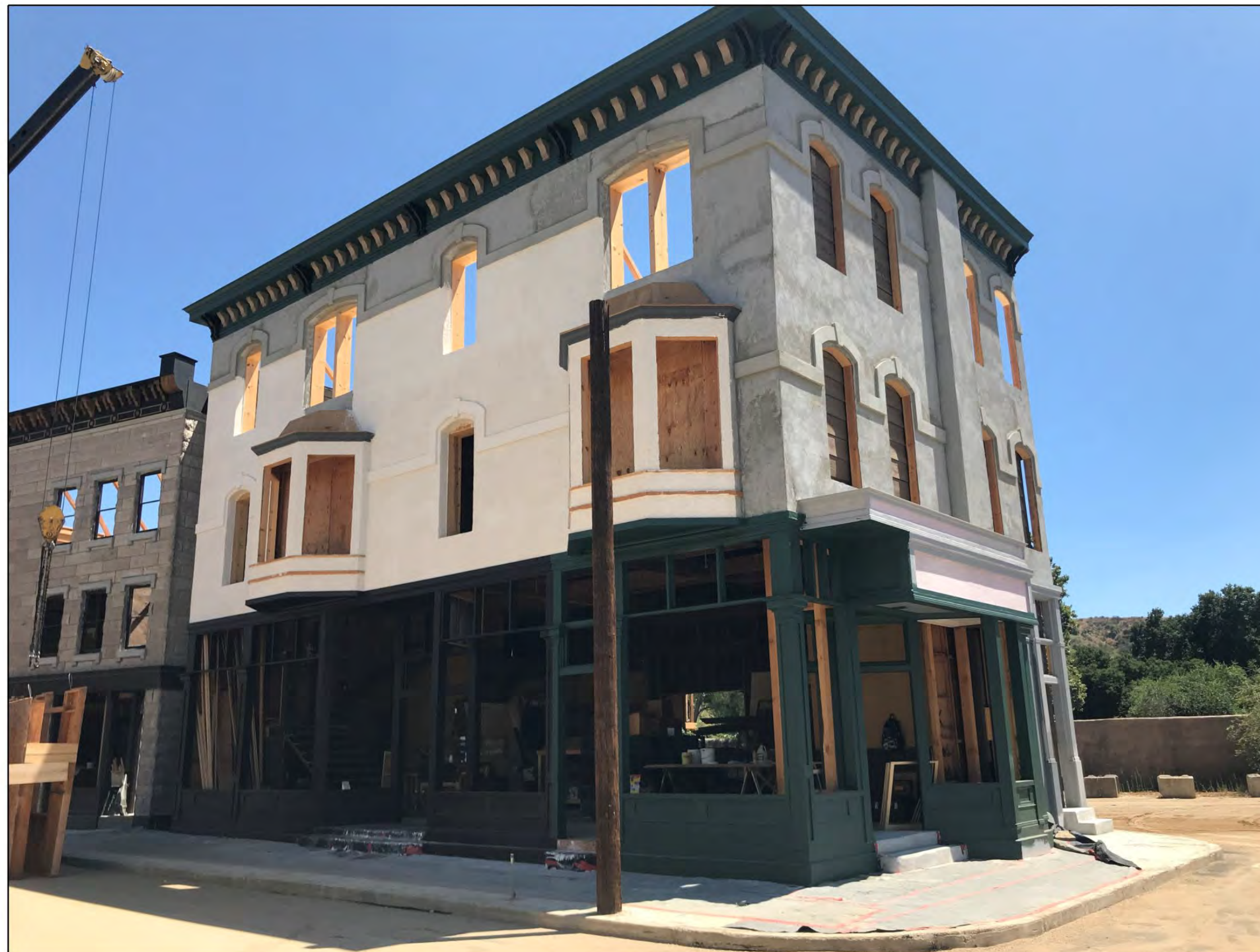
Part way through construction
