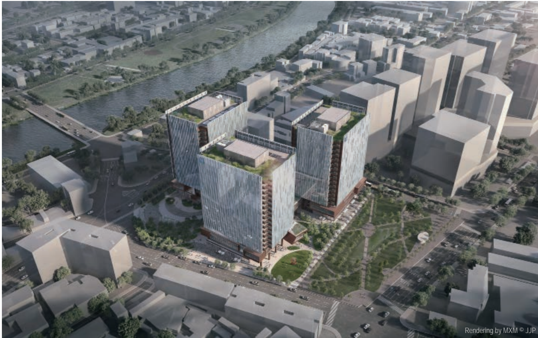
A new commercial campus with complex surroundings
