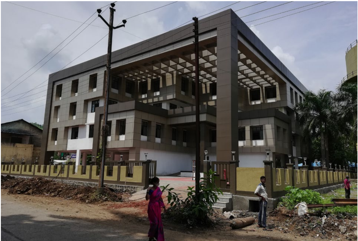
Post Completion View
