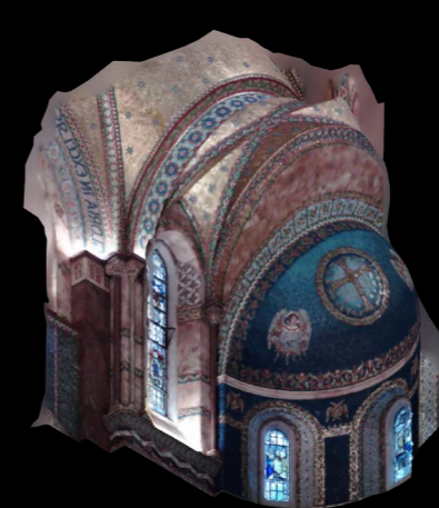
Quadripartite Ribbed Vault with Dome
