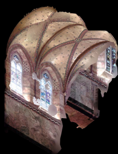
Quadripartite Ribbed Vault + Lateral Round Arches
