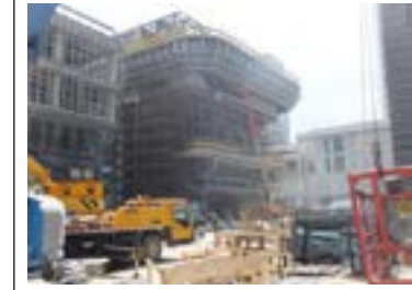
CONSTRUCTION PROGRESS ON STEEL FRAME Foster + Partners
