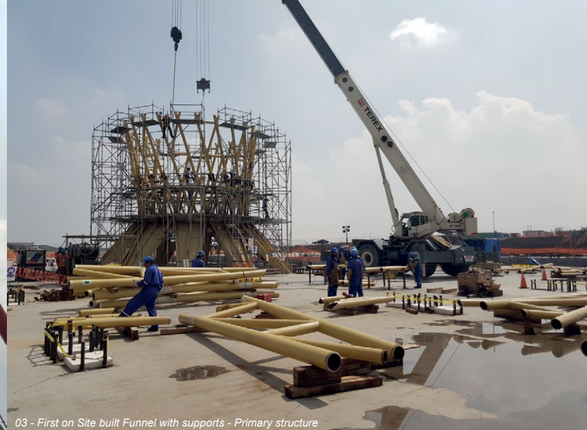
03 - First on Site built Funnel with supports - Primary structure
