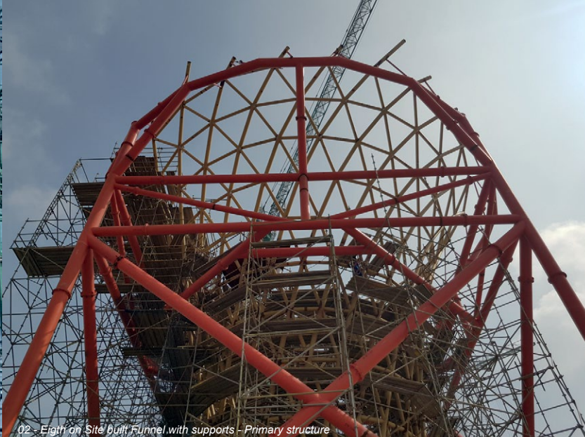
02 - Eighth on Site built Funnel with supports - Primary structure
