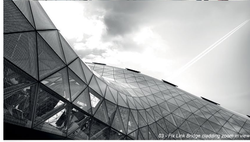
03 - Fix Link Bridge cladding zoom in view
