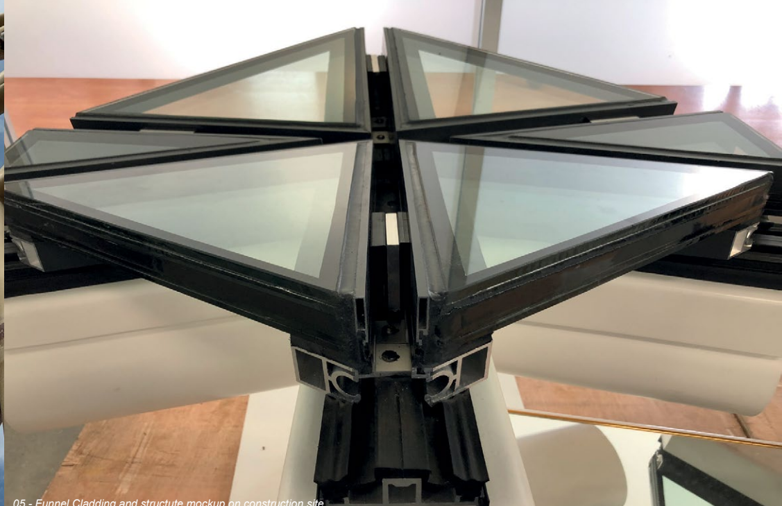
05 - Funnel Cladding and structure mockup on construction site
