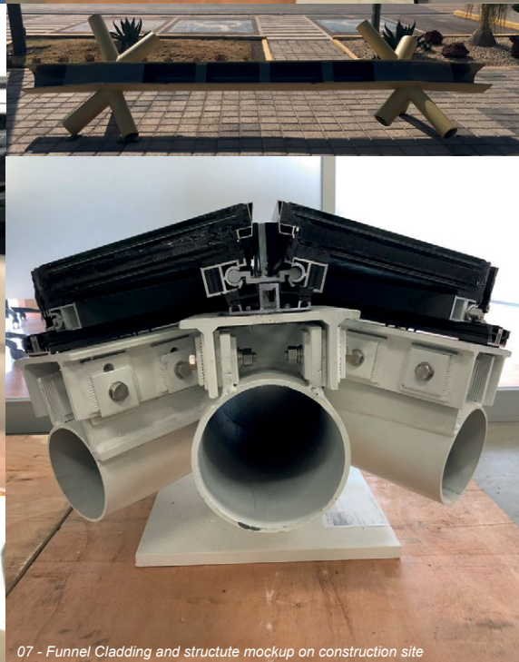
05 - Funnel Cladding and structure mockup on construction site
