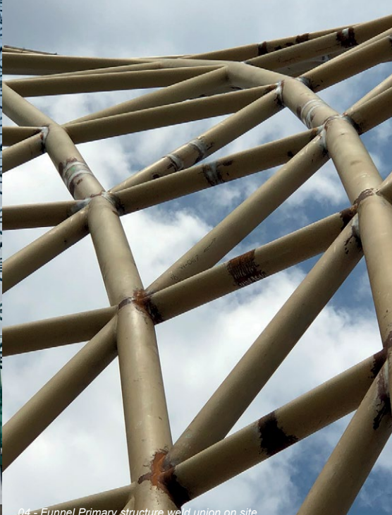
04 - Funnel Primary structure weld union on site
