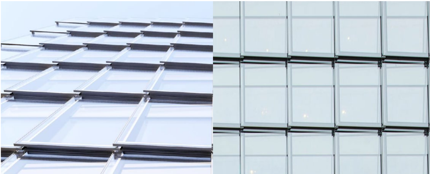
(up) Southern shingled "double-skin" facade, which balances high transparency with energy efficiency in its closed-cavity composition of glass panels. The materiality of glass is further animated by shingling the panels and the visual effect of overlapping overhangs. (Rhino, Enscape)
