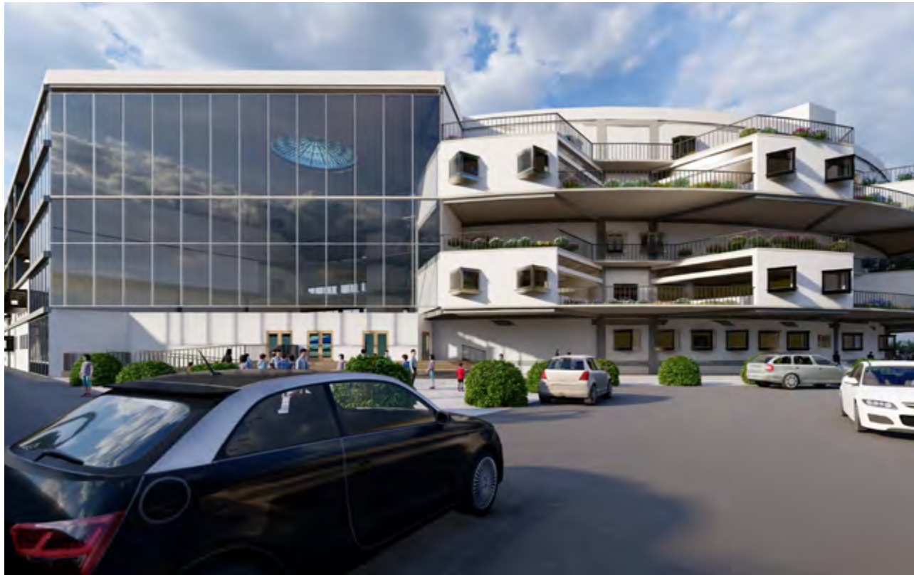
Discovery Center Main Building
