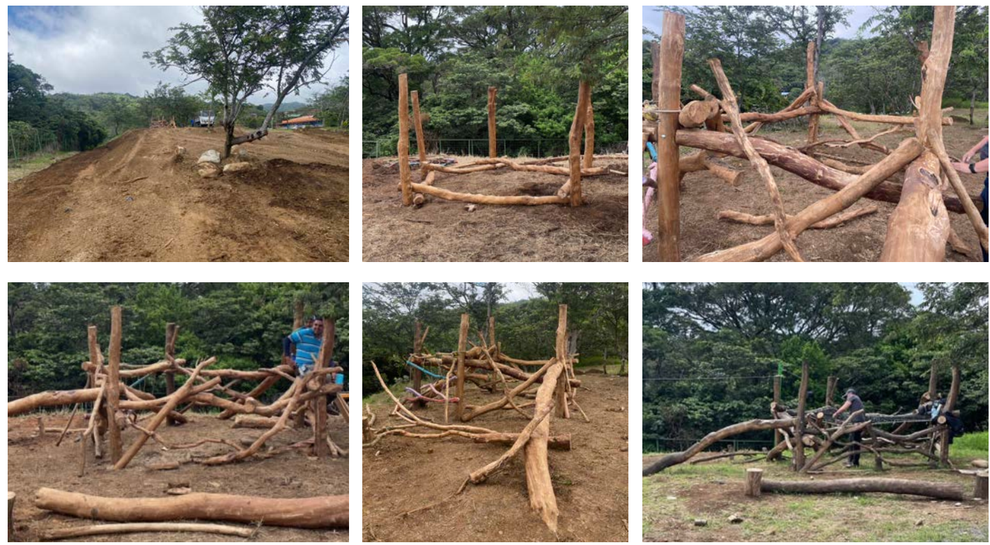
Construction process photos
