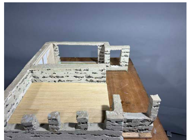
Townhouse sectional model: Pre-fabricated rock wall casts, with integrated wall joists for interior walls. Large aggregates are poured into the cast, along with stratified layers of strong mortar, creating the structural outer walls. The outside-facing mold is then removed, leaving behind a thick, self-insulating stone wall, and interior wall joists, ready for drywall. The system aims to cut down on the need for insulation means and labor.
