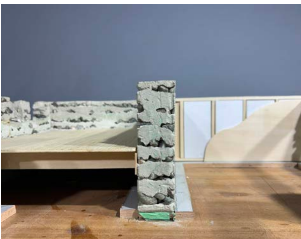
Townhouse sectional model: Pre-fabricated rock wall casts, with integrated wall joists for interior walls. Large aggregates are poured into the cast, along with stratified layers of strong mortar, creating the structural outer walls. The outside-facing mold is then removed, leaving behind a thick, self-insulating stone wall, and interior wall joists, ready for drywall. The system aims to cut down on the need for insulation means and labor.
